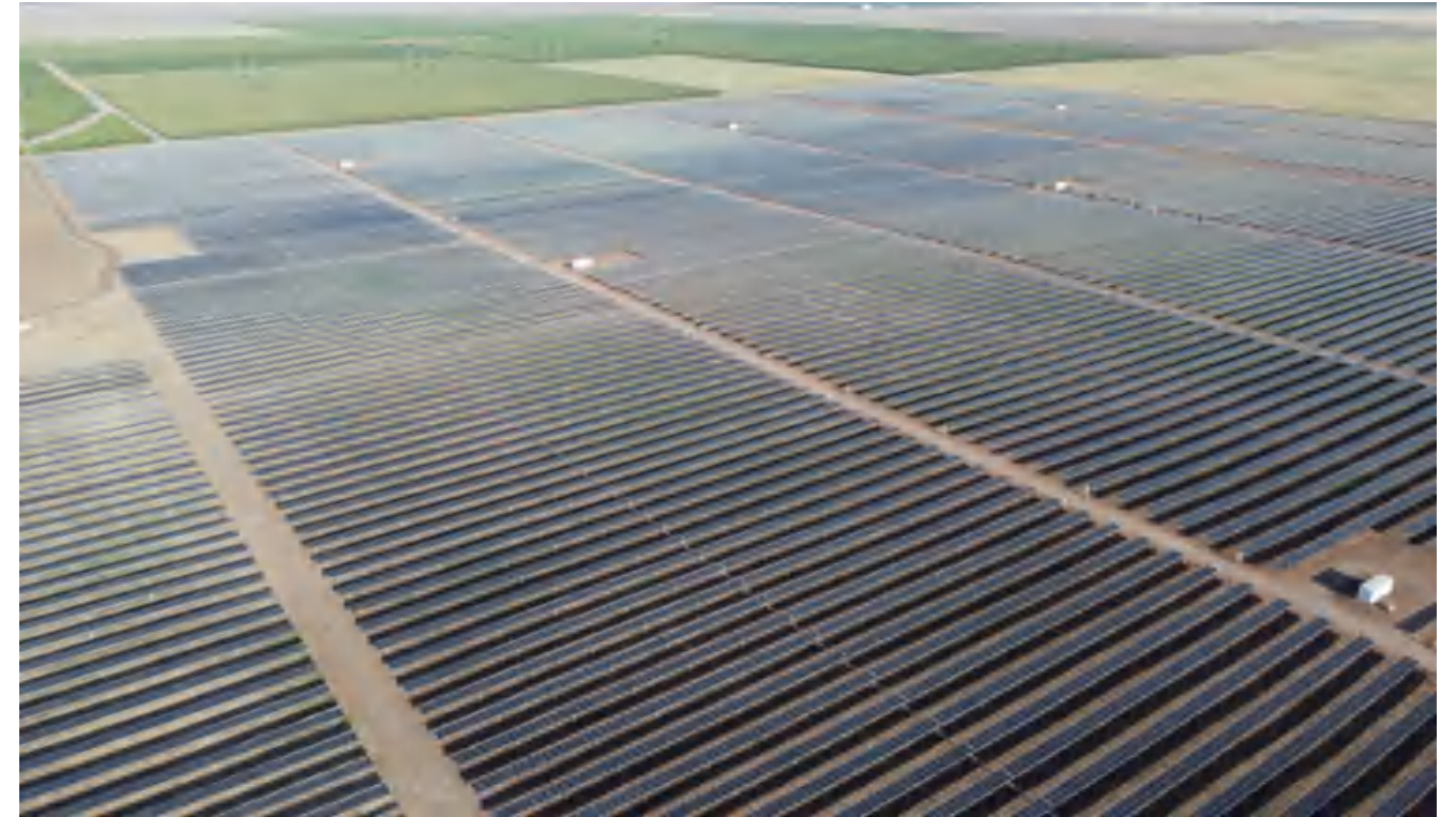
• 73 MWp Tulare County, California, USA
